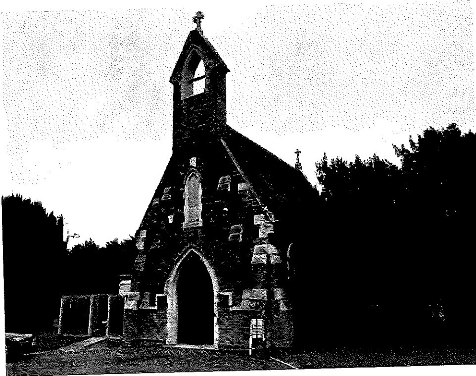
Main front elevation view from right hand side
